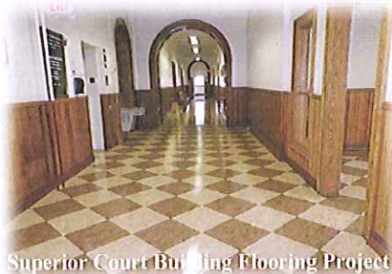
Superior Court Building Flooring Project
