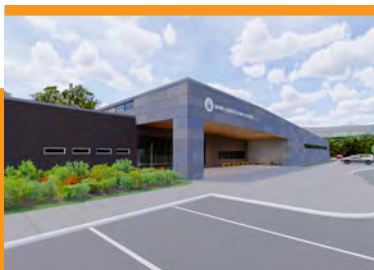
MAINE CORRECTIONAL CENTER
